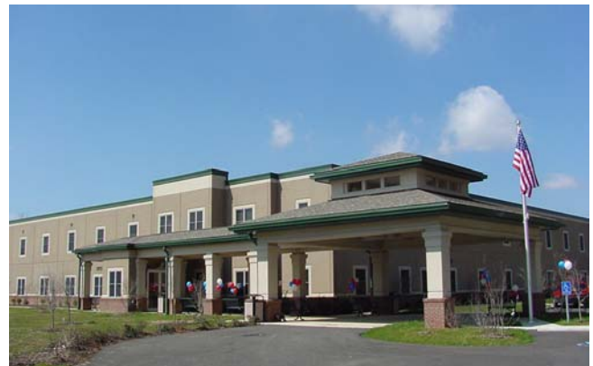
Eastern Kentucky Veterans Center, Hazard, Kentucky
